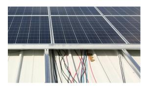
Over decades, cables and wires of solar and photovoltaic systems are exposed to various stresses, such as UV radiation, weather, mechanical influences, or even rodent bites and insect attacks.
